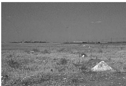
Figure 9. Course of the Villamalea qanat (Alcalá de Henares, Madrid) indicated by breather caps
