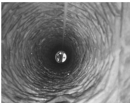
Figure 6. Breathing well. Fuente del Berro qanat
