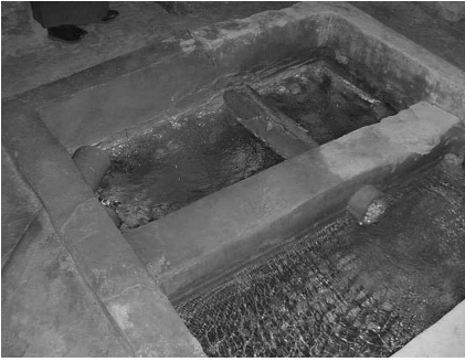
Figure 17. Main drain. Ocaña qanat
