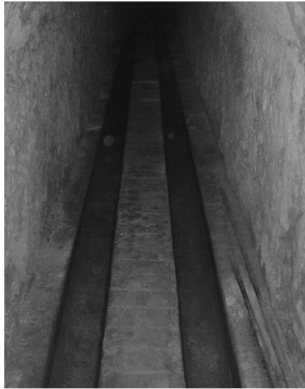
Figure 21. Conducting gallery with two channels carrying hard and soft water. Ocaña qanat
