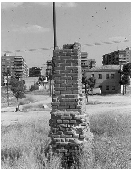
Figure 8. Breather. Alto Abroñigal qanat
